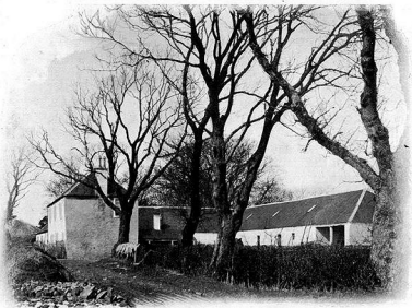
MOSSGIEL AT PRESENT.
