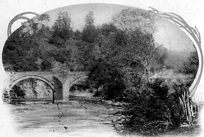
THE HOWFORD BRIDGE.
