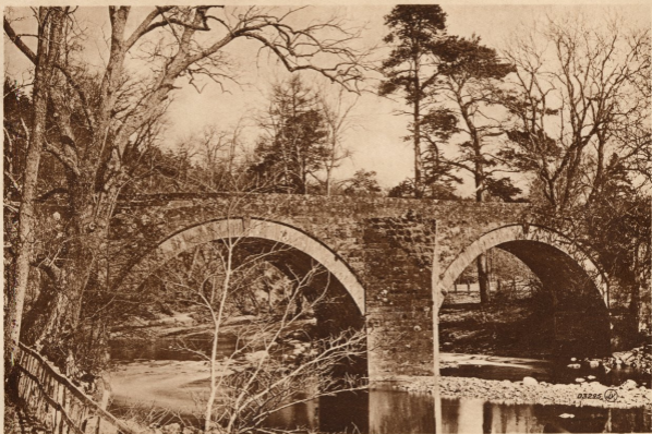
HOWFORD BRIDGE, NEAR MAUCLINE
