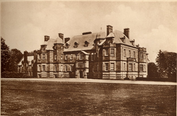
BALLOCHMYLE HOUSE (FRONT VIEW)
