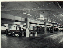
VIEW OF A FLOOR OF BUILDING No. 4.
